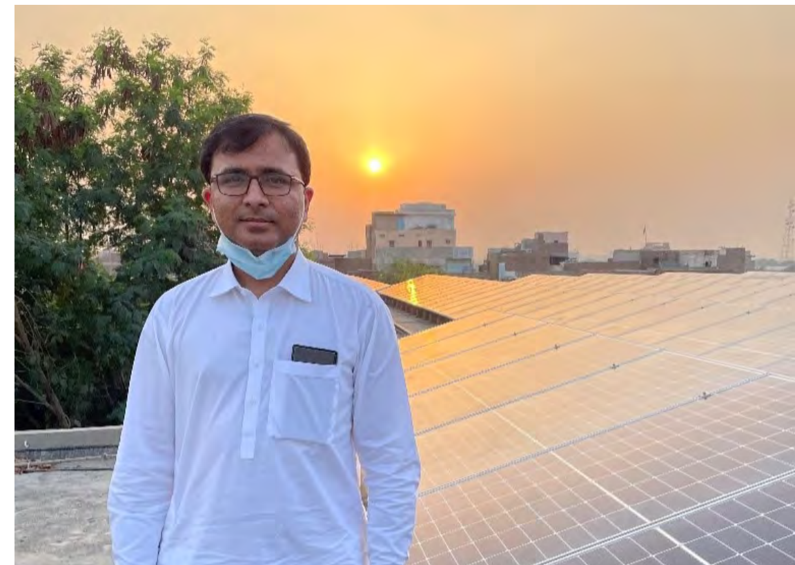
Project Director for Sindh Solar Energy Project by the rooftop solar installation on the Civil Hospital in Hyderabad
