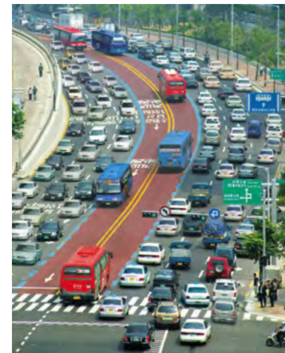
Median Bus Lane
